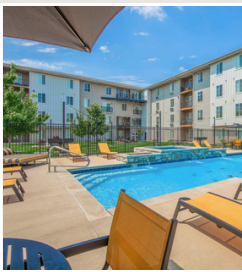
Trails Bend Apartments South Springfield
