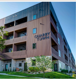
Quarry Town Apartments East Springfield
